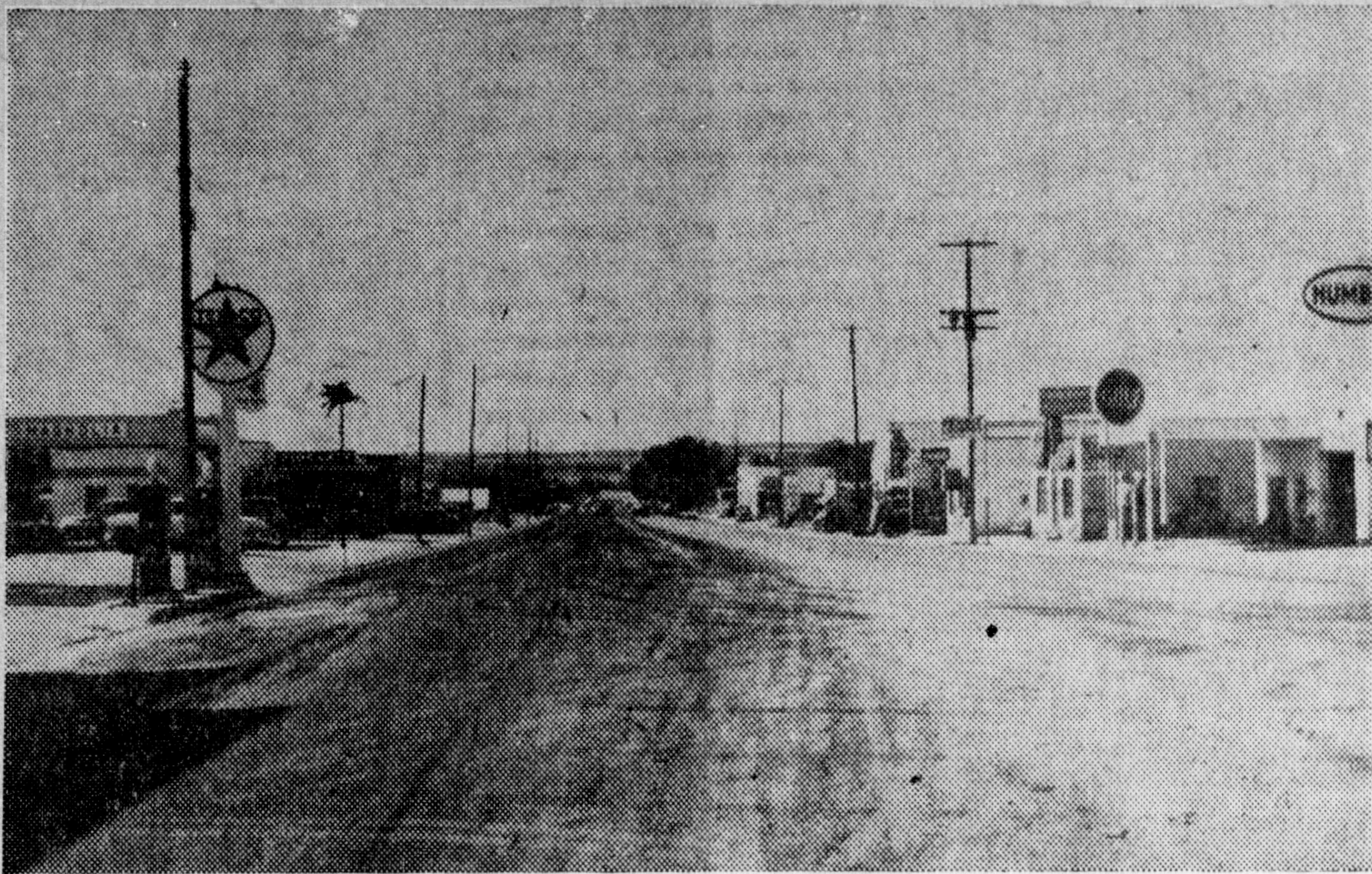
ALL FINISHED—Final touches have been applied and detour signs removed on South Main. The new, wide, curbed street, as seen from the Square, gives Highways 201 and 199 the best city entrance road in north Texas. —Mixon Studio Photo
